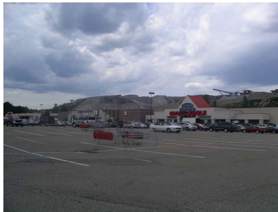
A Slag Dump near Pittsburgh has been redeveloped and is now a shopping center.
